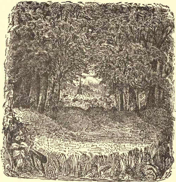
CENTRE REDOUBT ON HAVER ISLAND, OPPOSITE WATERFORD.
